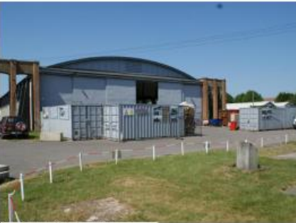
May 2023 Hangar 4 near elevations from east
