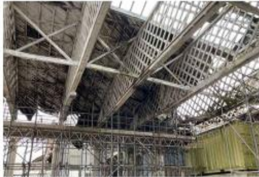
Belfast trusses remaining in-situ
