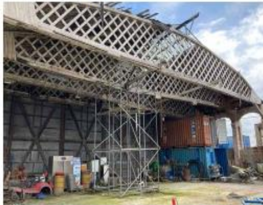
Belfast trusses and hangar doors remaining in-situ
