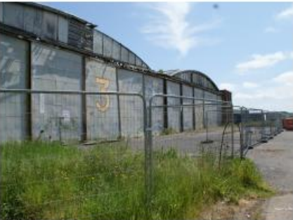
May 2023 Hangar 3 southern elevation
