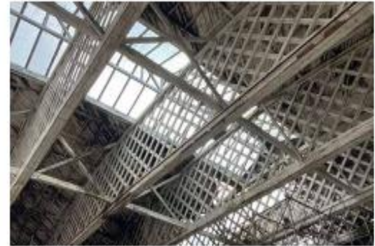
Section of remaining rooflight
