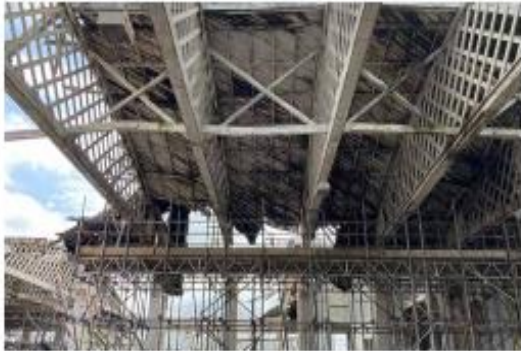
Belfast trusses remaining in-situ
