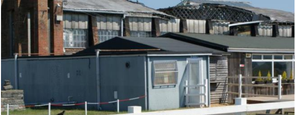
From the south - single storey buildings are generally post 1980. The former Flight Commanders office is to the right - see subsection 8 for fuller description of this building.
